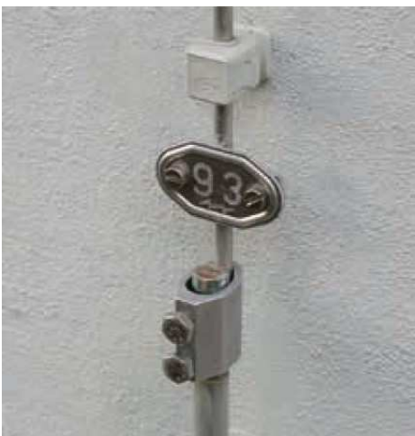
Test Joint with Number Plate
