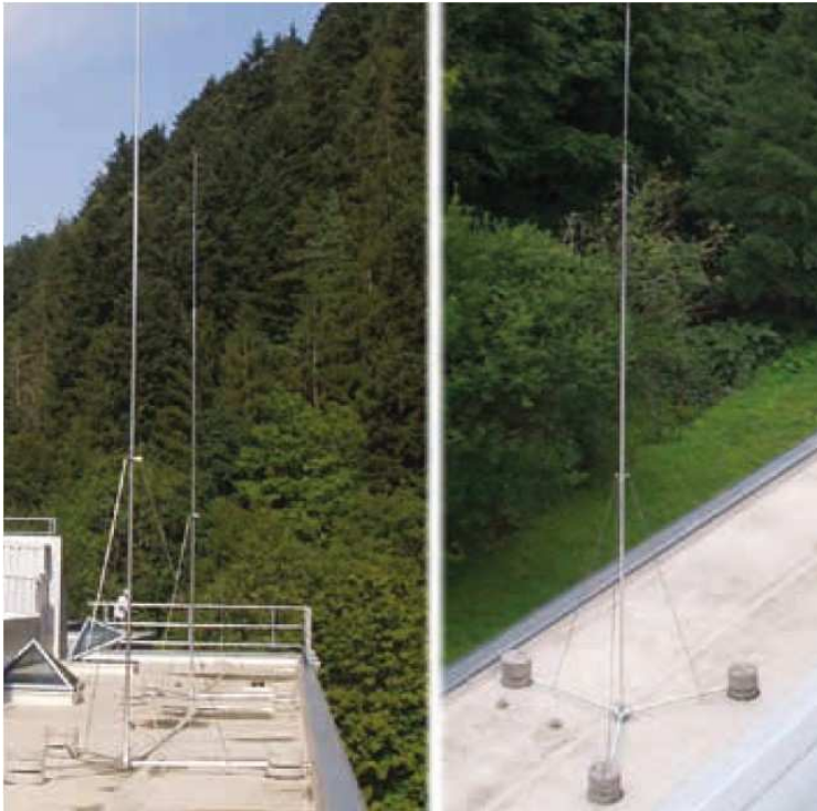
Self-supporting Air-termination Rods with tripod
