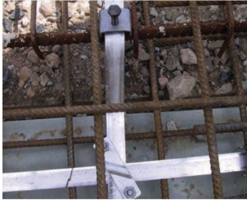
Foundation earth electrodes in the concrete reinforcements
