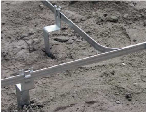
Foundation earth electrodes (strips)
