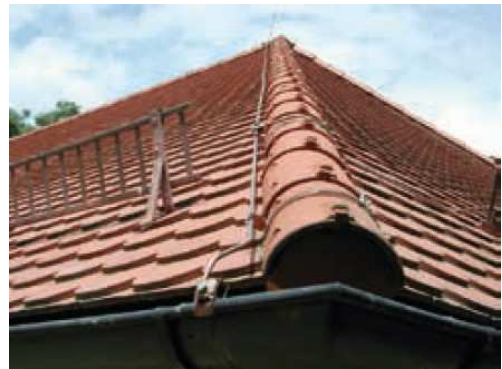
Air-termination system with connection to gutter
