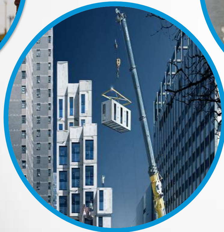
Fabrication & Modular Construction 预制&模块化建造
