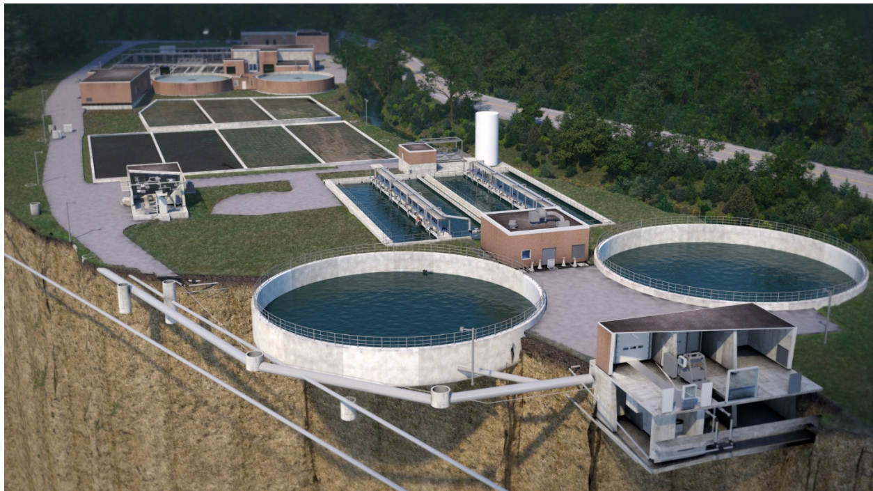
Pleasant Hills Authority – SSO Elimination Project
