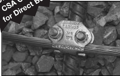
Wire to Rebar
