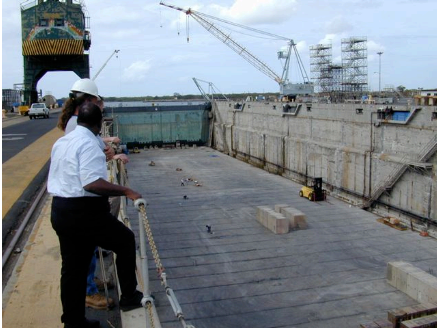
Dry Dock rehabilitation Pearl Harbor
