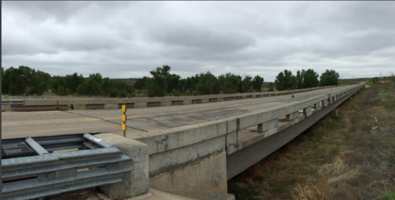
Sierrita de la Cruz Creek Bridge, Amarillo, Texas Constructed in 2000
